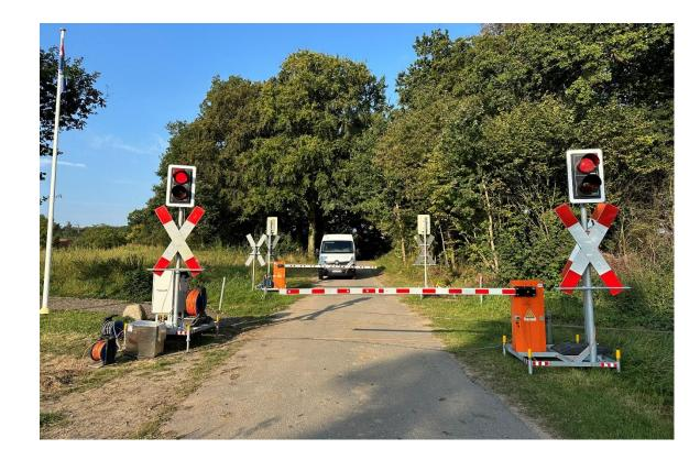
> The automatic temporary protection of a level crossing with axle counting technology
